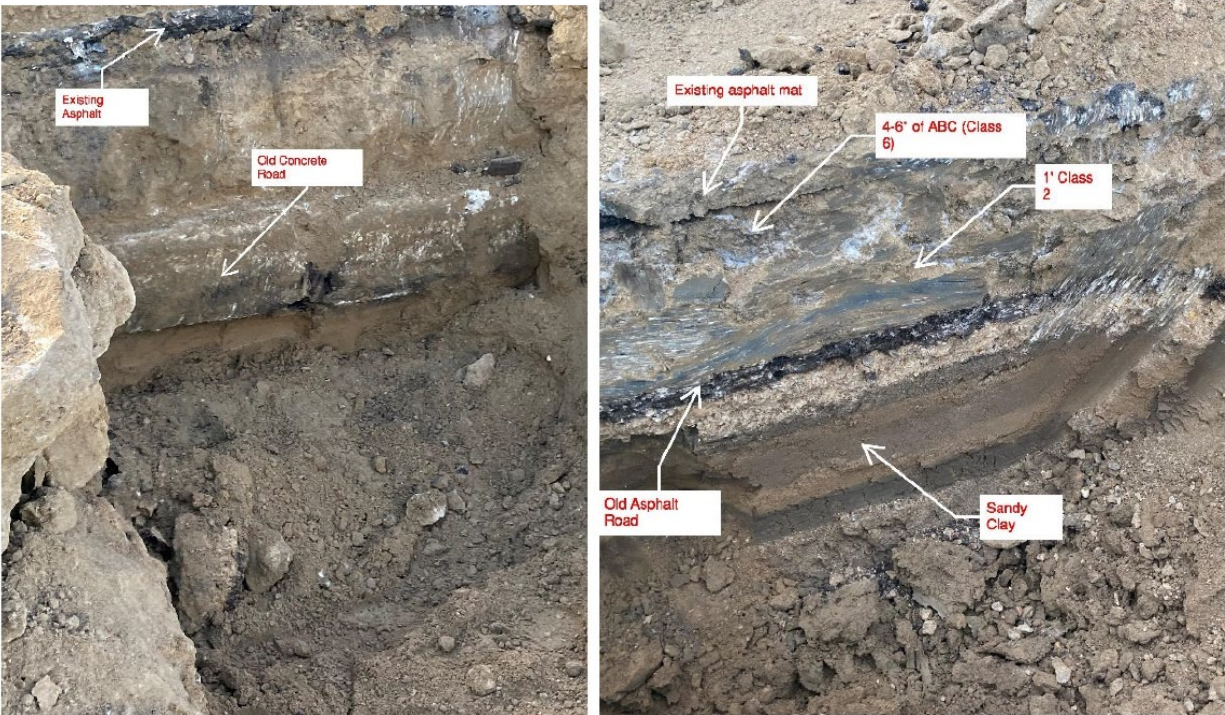
Figures 3 and 4: Exposed cross section of existing US34 prism showing buried roadway.
