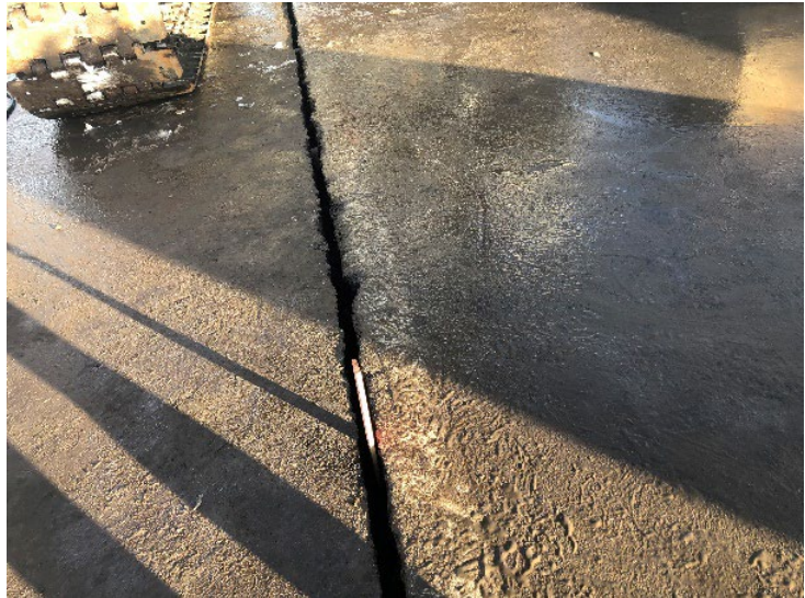
Figures 1 and 2: Cracking resulting from erosion and differential settlement between the shoulder and through lane.
